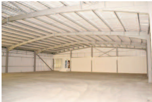
1 ST FLOOR MAIN HALL – VAULTED
