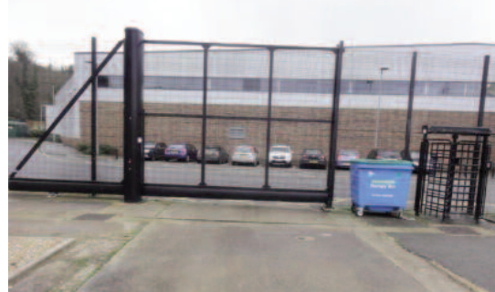
REAR VEHICLE & PEDESTRIAN SECURITY GATES
